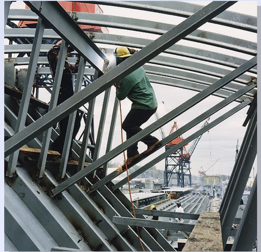
Building a barge in a large shipyard
